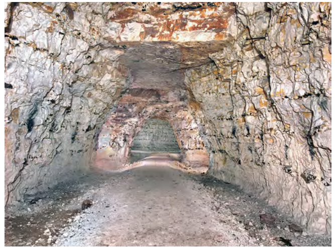
One of the unlined chalk galleries in the Scout mine.
